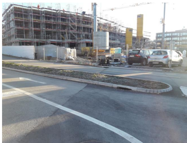
Figure 4 - Chantier Epinettes Source : TPF
