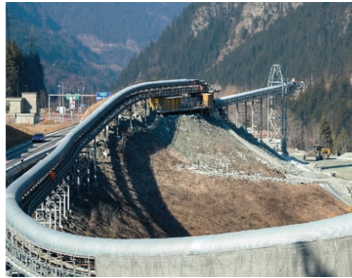
At the northern portal in Göschenen: the conveyor belt for the excavated material during construction of the second Gotthard road tunnel.
