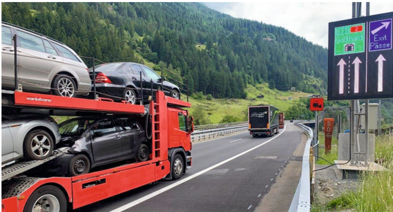
The extended exit lane on the Gotthard stretch near Göschenen (canton of Uri).
