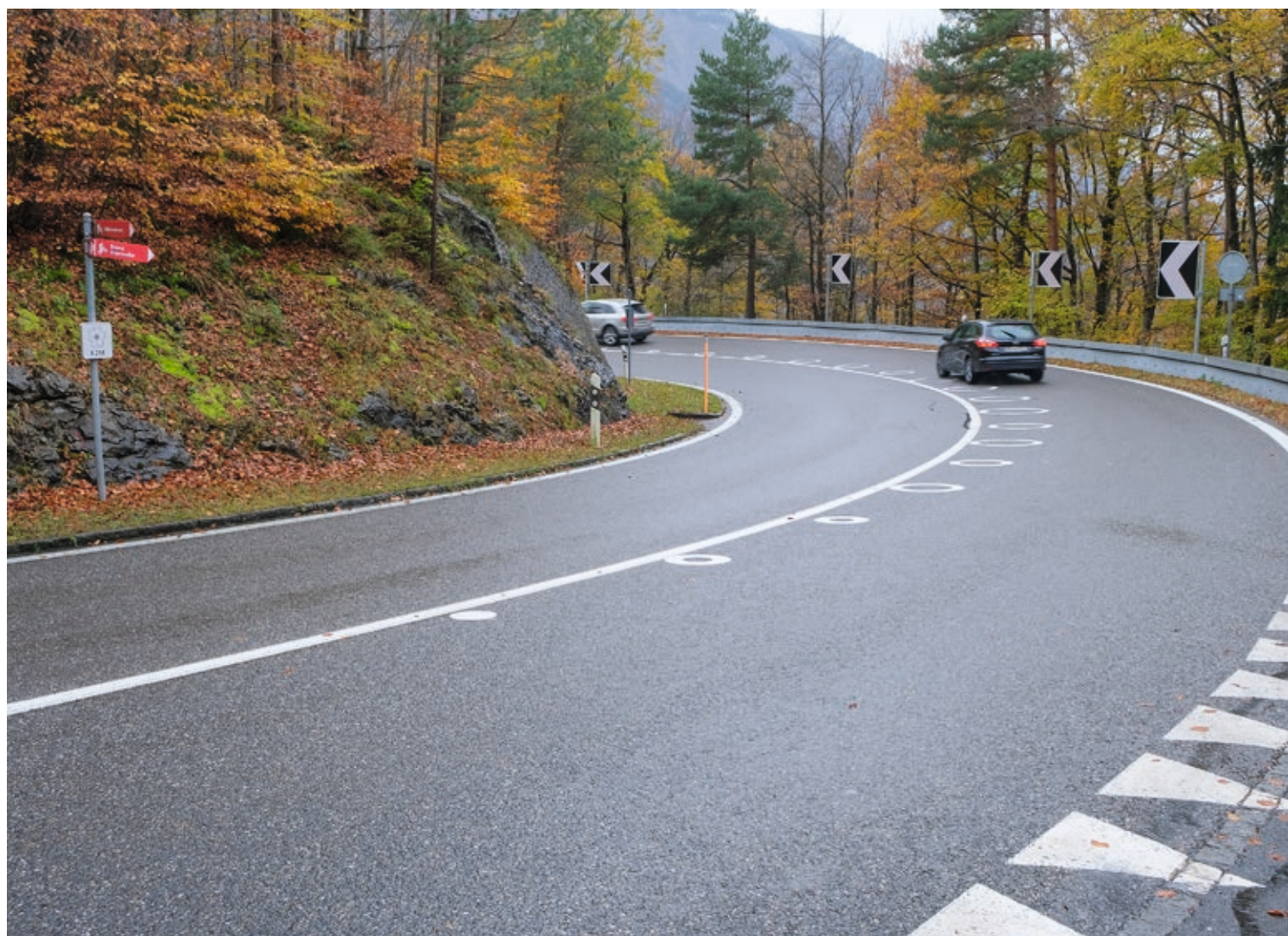
Special circle markings to improve road safety on the Brünig pass.
