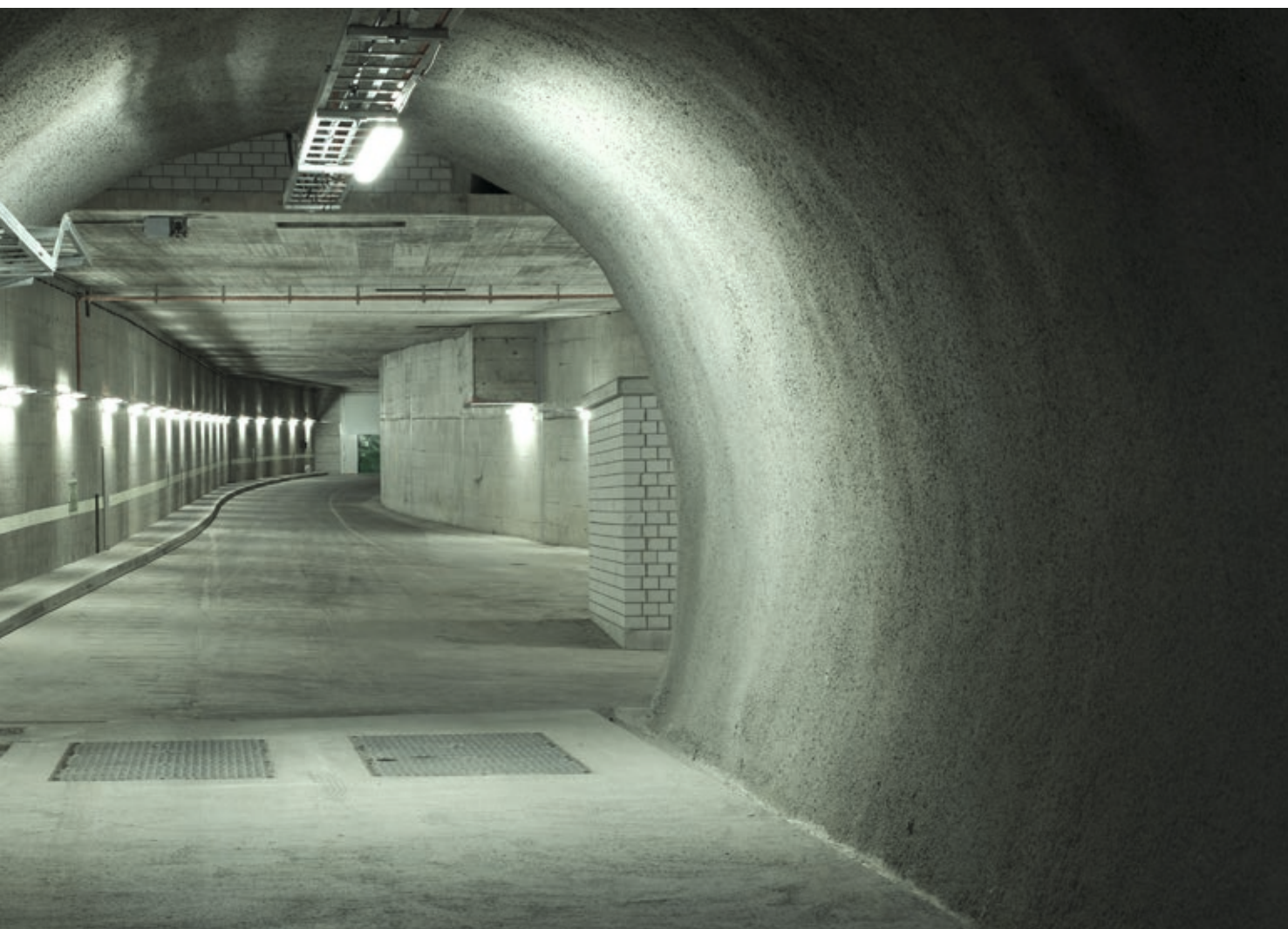
The safety gallery at the Milchbuck tunnel in Zurich.
