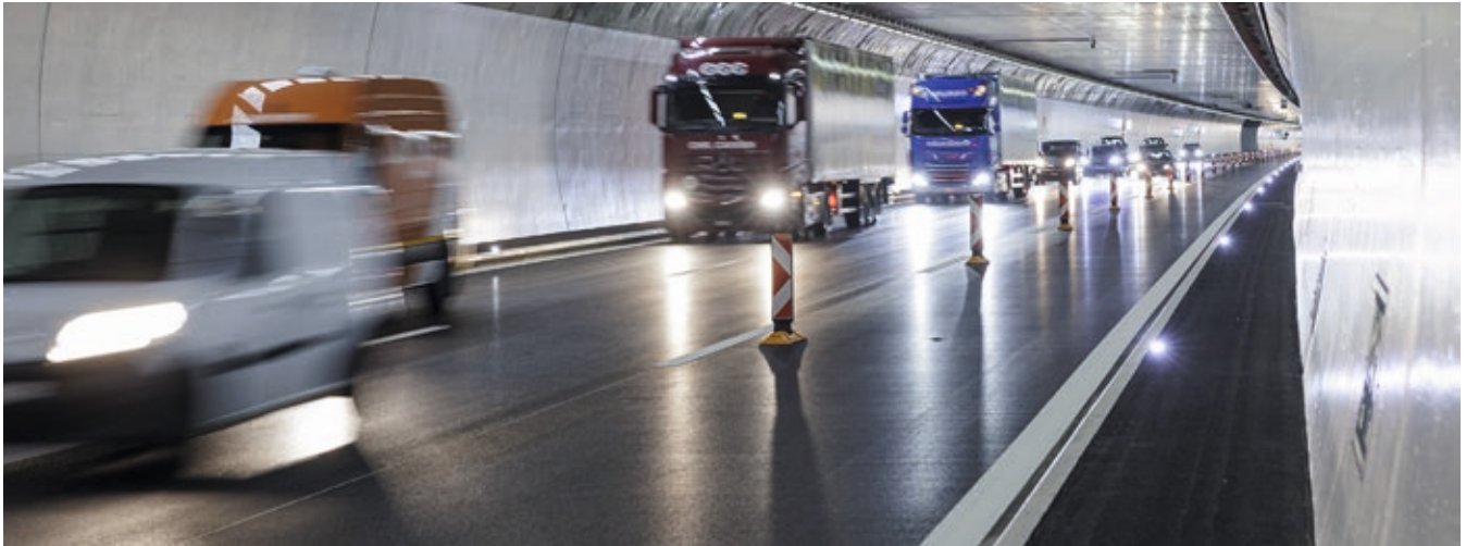
The third tube of the Gubrist tunnel near Zurich was opened in April 2023.
